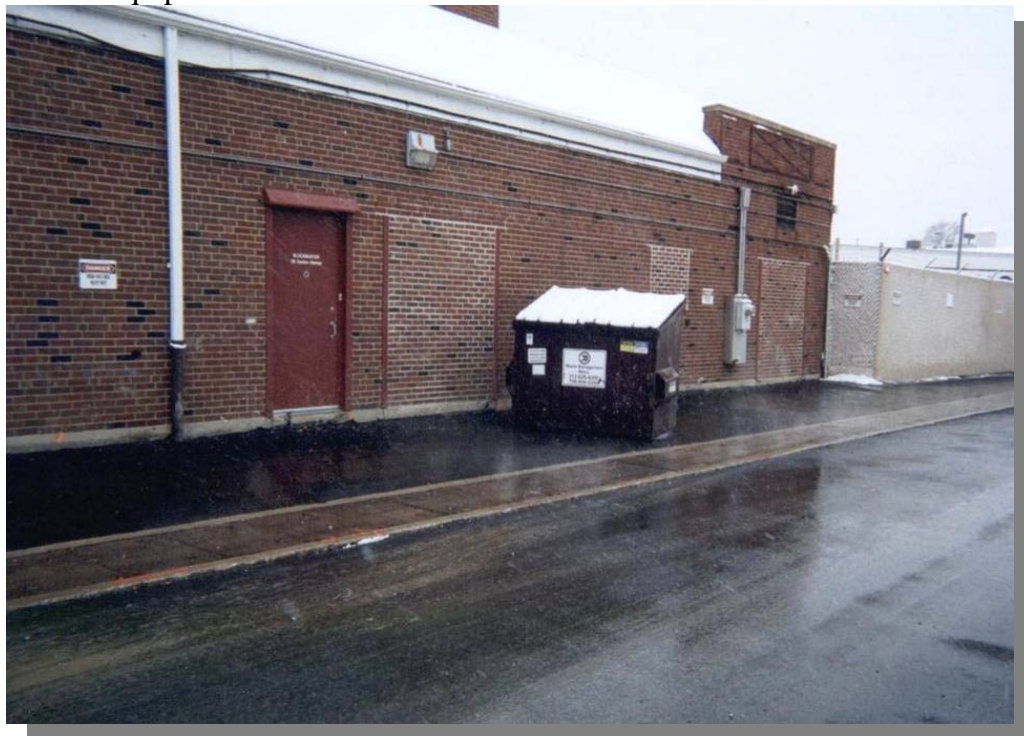
Figure 5: ERH system in operation behind a dry cleaner in a strip mall in suburban Chicago. ERH is keeping alley clear of snow and equipment is hidden behind chain link fence.
